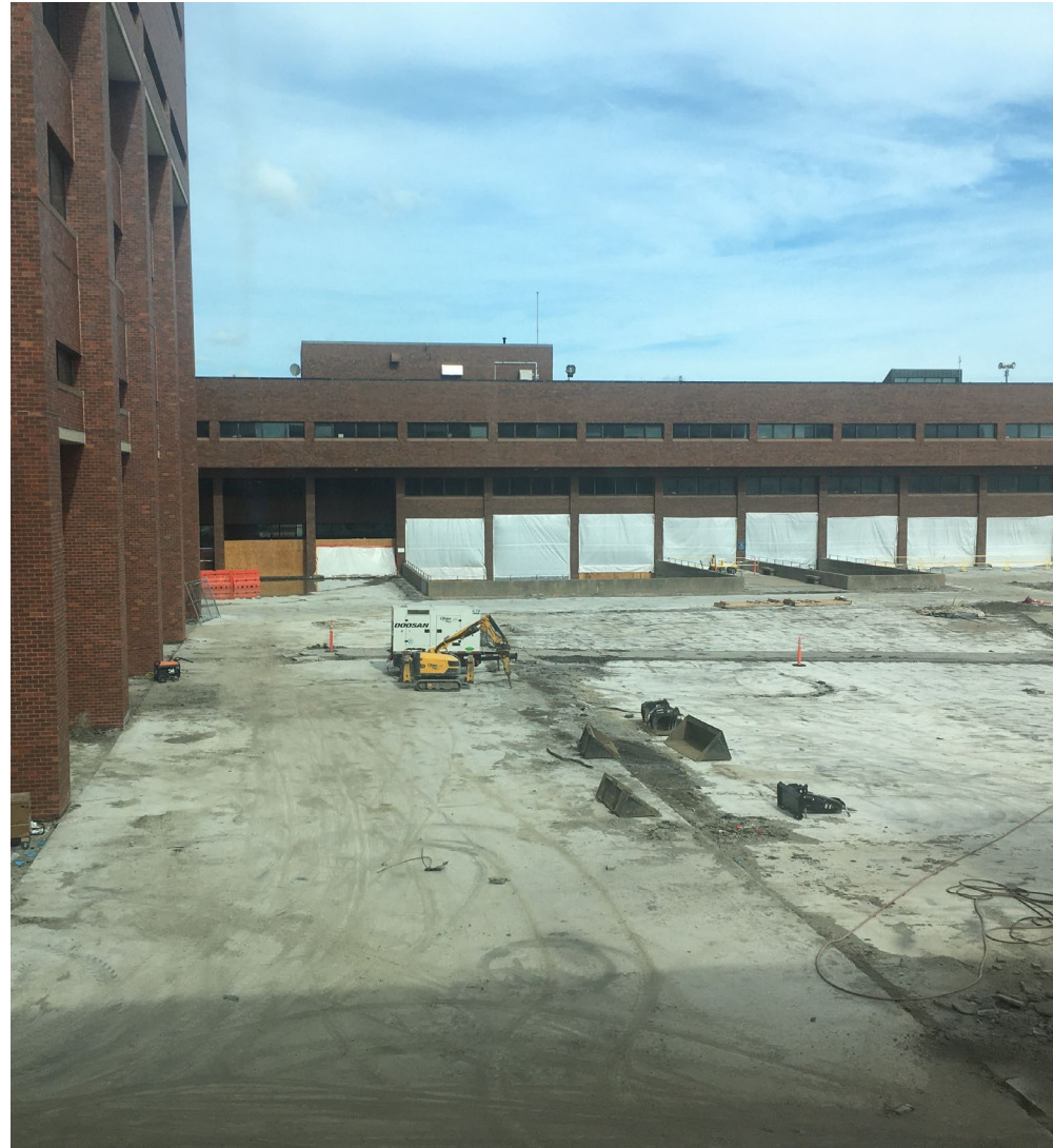
Plaza with pavers and waterproofing removed
